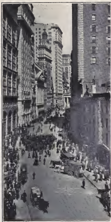
THE BROAD STREET CANYON Showing curb market in operation
