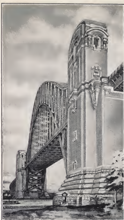
HELL GATE BRIDGE
