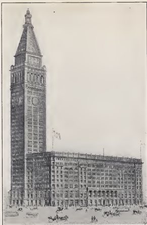
METROPOLITAN LIFE BUILDING
